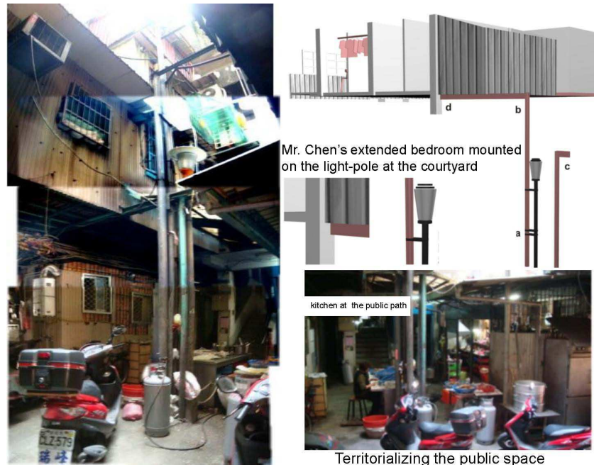
Figure 5 Metal-sheet rooms mounting on the pole trunk at the center of the designated public domain.
